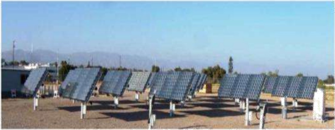
Fig. 25. Installation at the University of Northridge, California, June 2010
