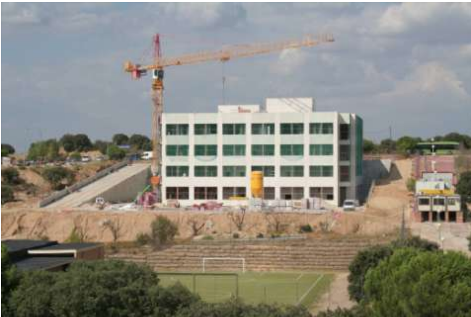
Fig. 22. CTB Construction. 2010 Status report.
