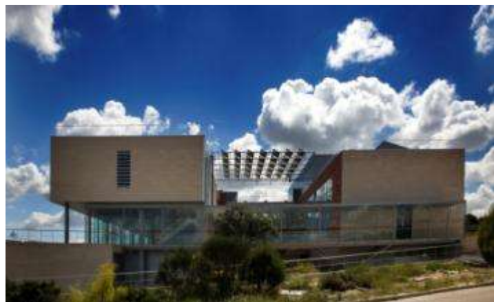
Fig. 30. Side view of CEDINT building in Campus Montegancedo
